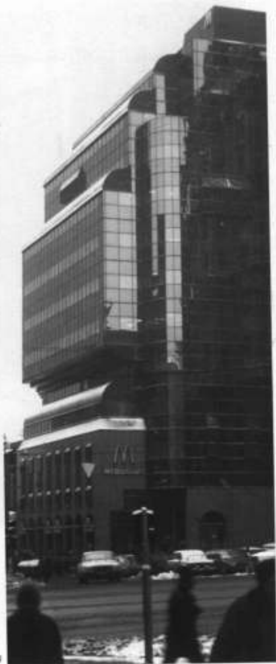
■ McDonald's Building, Gazette Alley, 1993
